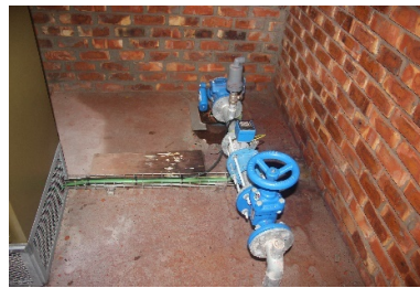
Borehole GWA5C in Kwanokuthula
