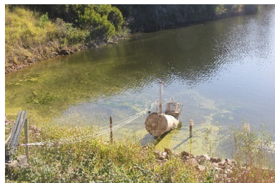
Intake at Roodefontein dam
