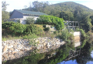
Keurbooms raw water PS and inlet works
