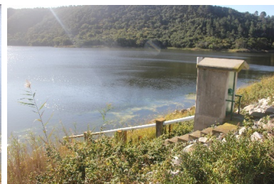
Level indicators at Roodefontein dam
